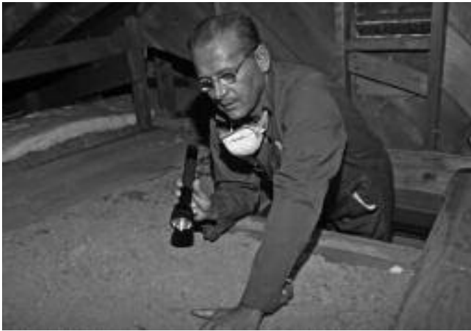
Attic insulation inspection – SALEM ELECTRIC
